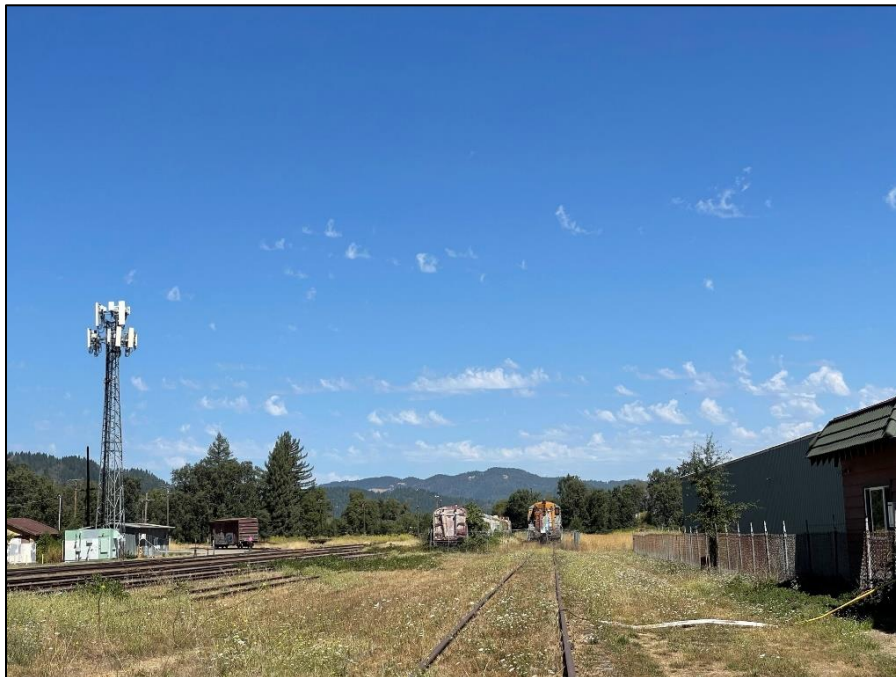
View facing north along railyard
